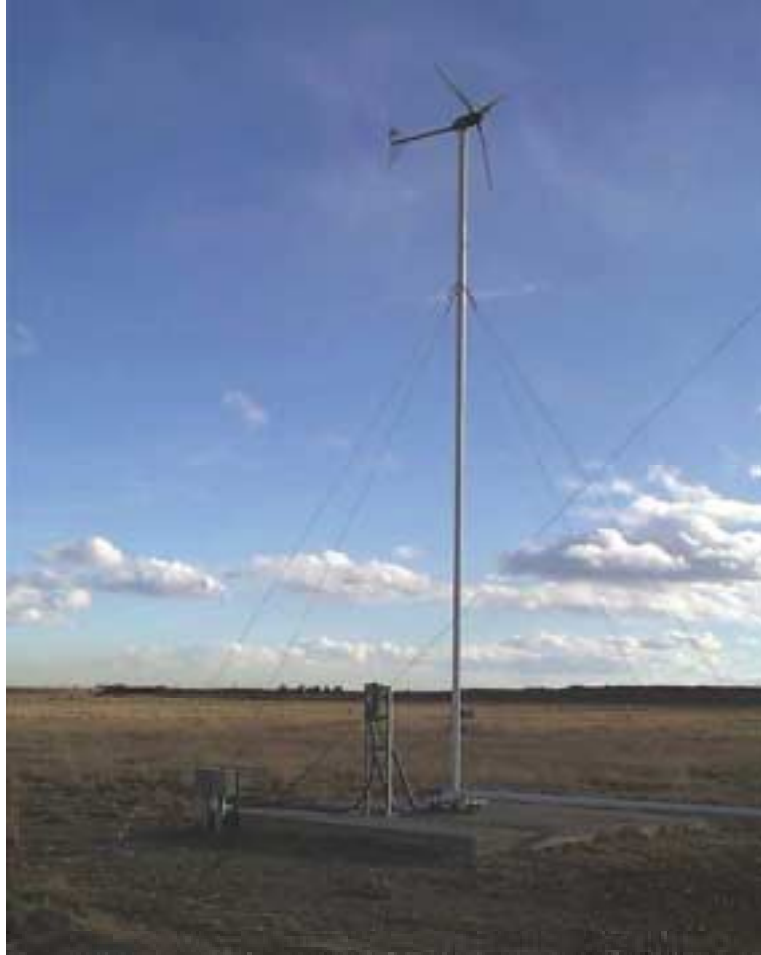
Figure 1. Whisper H40 turbine at the NWTC test site.
