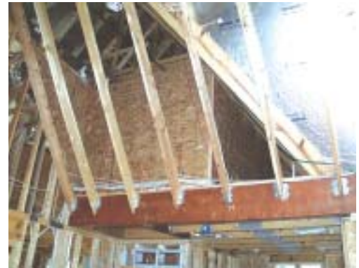
Child's loft utilizes unused attic space efficiently, but posed unique challenges in insulation and airtightness detail
