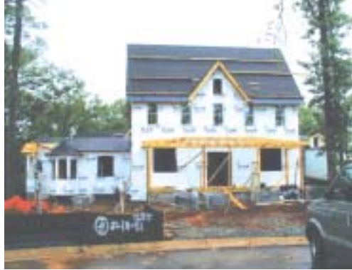
Strategy of well-integrated window and door flashing with housewrap
