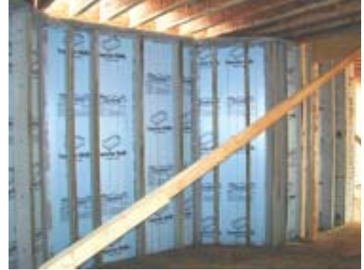
Superior wall system contributes to a very high performance home with overall R value of 24
