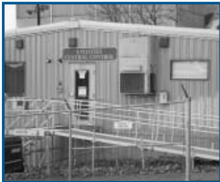
This building houses Weirton Steel's utilities central control room.
