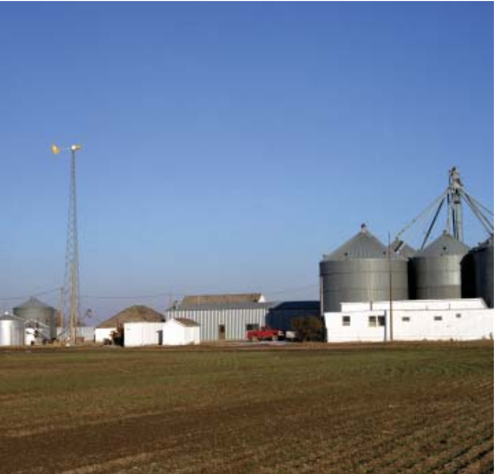
This 10-kilowatt Bergey wind turbine, installed on a farm in southwestern Kansas, produces an average 1700–1800 kilowatt-hours of electricity per month, reducing the owners utility bills by approximately 50%. Warren Gretz, NREL/PIX09614
