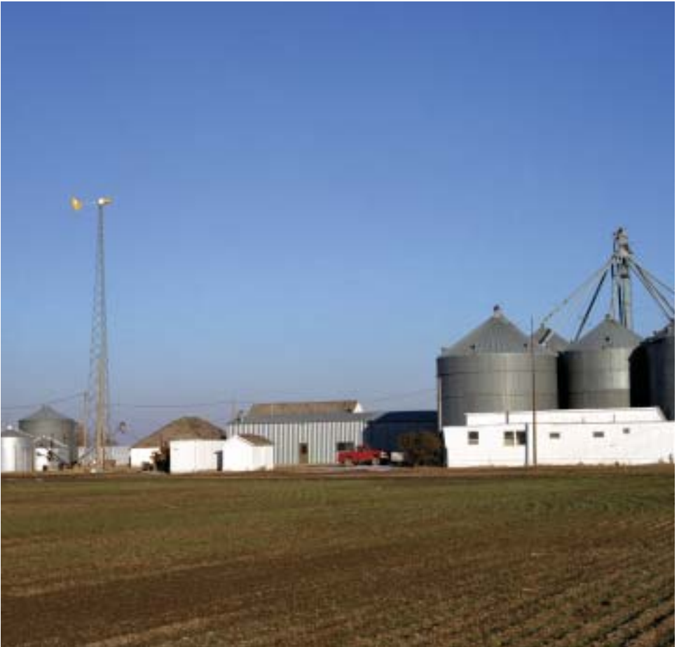
This 10-kilowatt Bergey wind turbine, installed on a farm in southwestern Kansas, produces an average 1700–1800 kilowatt-hours of electricity per month, reducing the owners utility bills by approximately 50%. Warren Gretz, NREL/PIX09614
