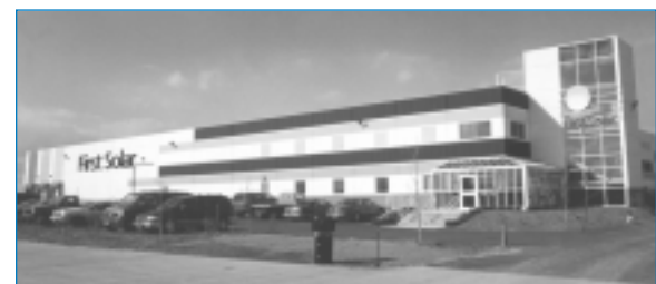
First Solar opened this high-volume PV manufacturing plant in Toledo, Ohio, in 2000. When fully operational, it is expected to produce 100 megawatts per year of thin-film, cadmium-telluride modules.
