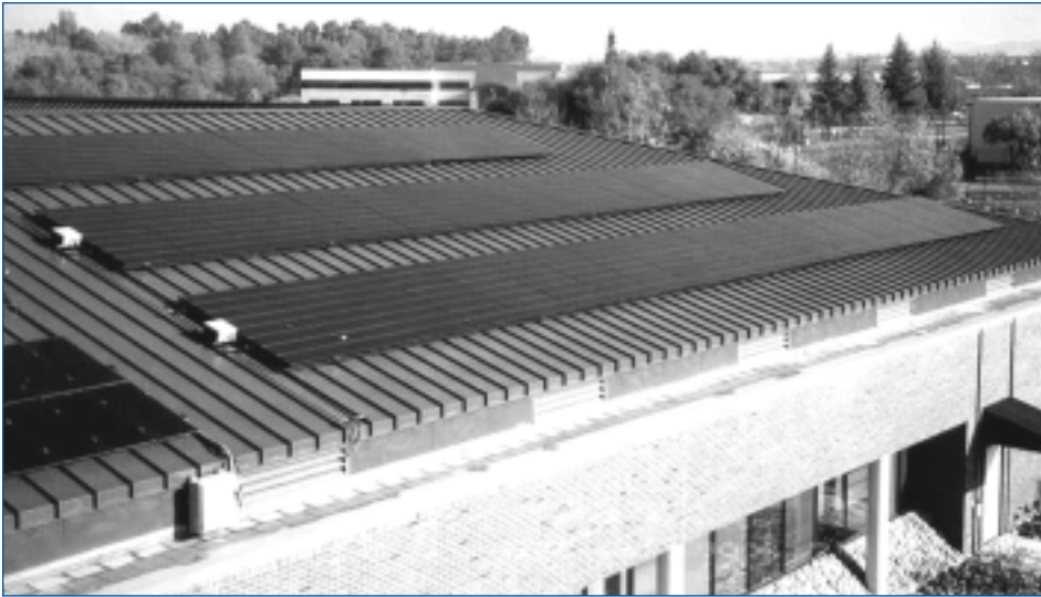
This 12-kilowatt (kW) array of CIGS thin-film modules is one of several systems sold by Siemens Solar Industries. The company is expanding its production line (the only one in the world for this material) from 700 kW per year to multimewatt-per-year production.
