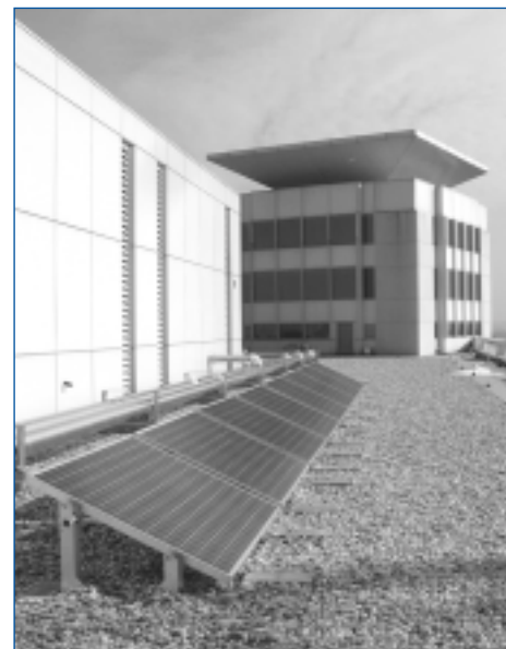
This 2.4-kW solar electric system installed on the headquarters of the Federal Energy Regulatory Commission produces 3,600 kWh of electricity per year that are used exclusively by this building.
