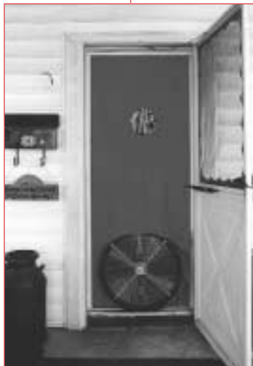
New Mexico crews use the blower door to identify and mitigate air infiltration.
