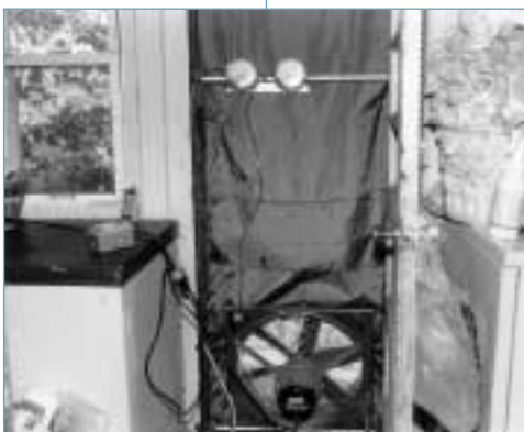
Nevada uses the blower door to identify and mitigate air infiltration.
