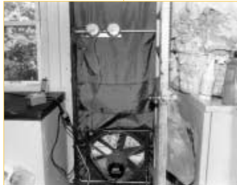
Mississippi crews use the blower door to identify and mitigate air infiltration.
