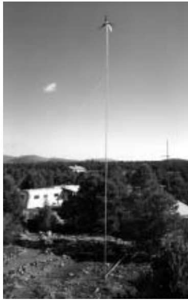
A Southwest Windpower Air 303, 300 watt turbine is the sole source of electricity for this remote home in northern Arizona.
