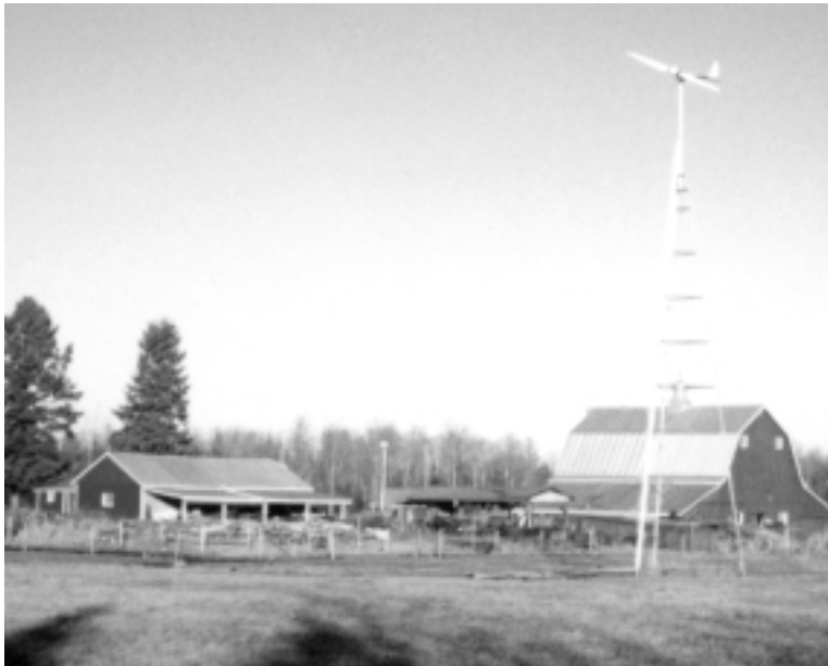
In Clover Valley, Minnesota, this 3-kW Whisper H175 turbine on a 50-foot tower is connected to the utility grid to offset the farm's utility-supplied electricity.
