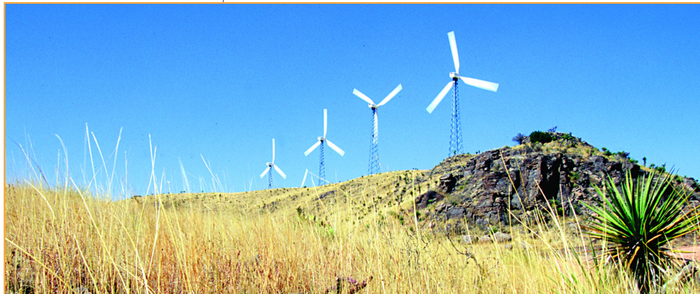
American Electric Power operates this demonstration wind power plant, rated at 6.6 megawatts (MW), near Fort Davis, Texas. The plant features new wind turbines developed by Zond Wind Corporation (now GE Energy Wind) of Tehachapi, California and developed with partial support of DOE's Wind Program.
