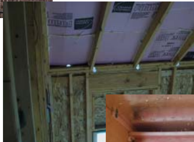
Superior Wall system featuring R-5 foam board insulation (exterior face) and R-19 batt insulation (wall cavities).
