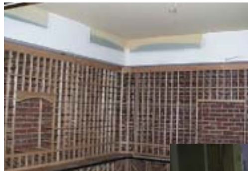
Conditioned wine cellar.
