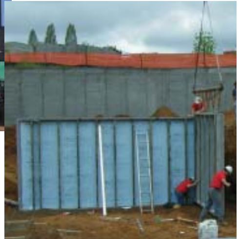
Superior Wall system featuring R-5 foam board insulation (exterior face) and R-19 batt insulation (wall cavities).
