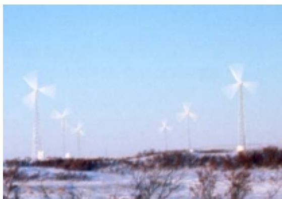
Figure 2. A 0.5 MW hybrid wind plant in Kotzebue, Alaska, provides power for a remote village.
