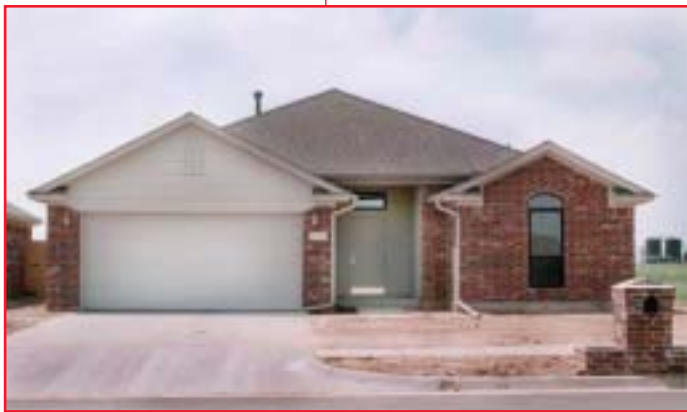
Home ventilation is improved by continuously mixing fresh air with recirculating interior air. Indoor air quality is substantially improved by virtually eliminating fumes from paints and adhesives during construction.
