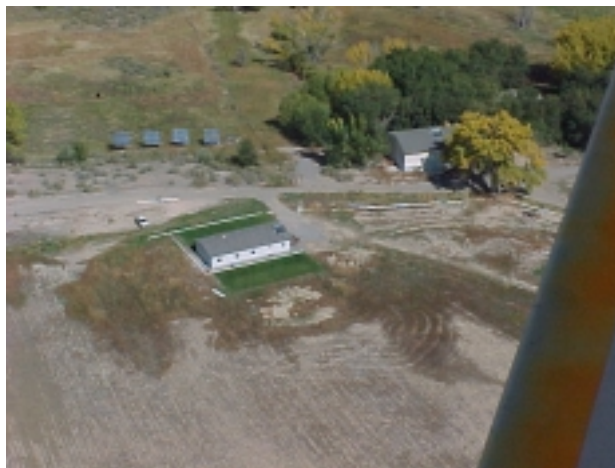
Aerial View of PV Arrays
