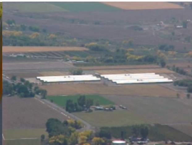
Aerial View of Galvanized Roofs
