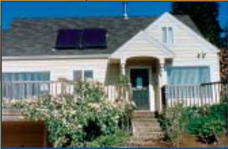
Photo courtesy of Eugene Water and Electric Board
