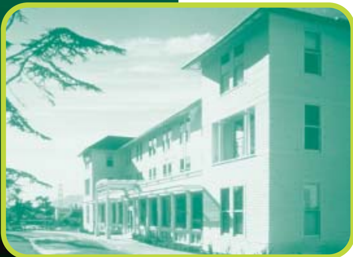
Thoreau Center for Sustainability, San Francisco Photo: Courtesy of the Thoreau Center
