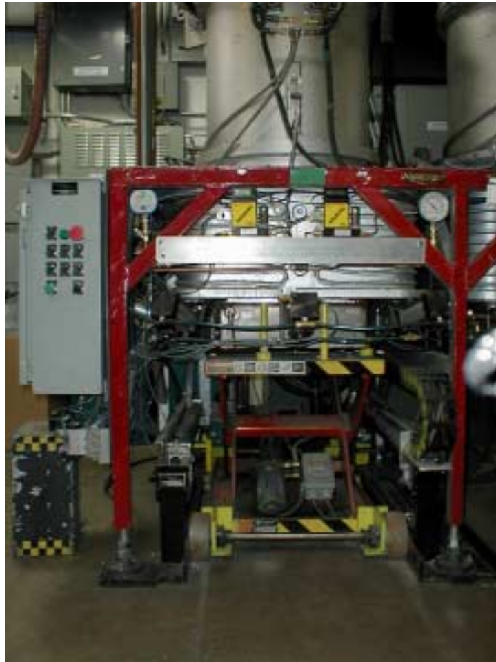
Figure 25 New Ingot Loading Cart – In Place
