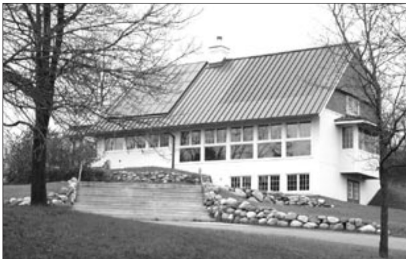
The recently completed “Nature House” at the Leslie Science Center in Ann Arbor, MI, is an environmental learning center that combines PV with other solar technologies. Features include a First Solar 2-kW solar-electric array composed of CdTe thin-film modules; solar thermal panels for heating water; windows designed for direct-gain sunlight in winter; and an 8-inch Trombe wall for heat storage. Energy-efficient features include compact fluorescent lighting and appliances.
