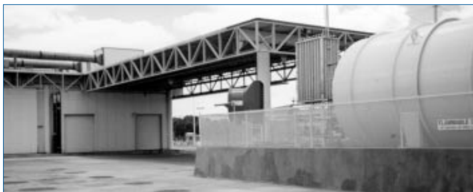
Figure 6. Northwest fueling station, showing canopy where fuel lines run from tank to fueling lanes
