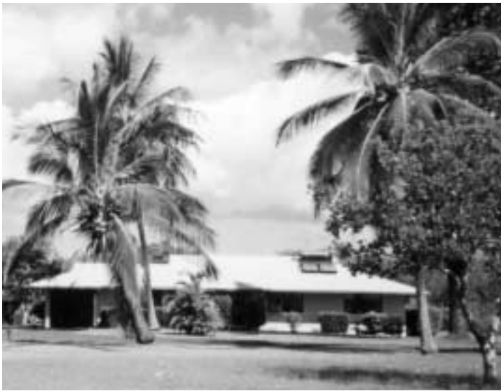
Solar water heaters on staff residences at the Pacific Tsunami Warning Center in Hawaii
