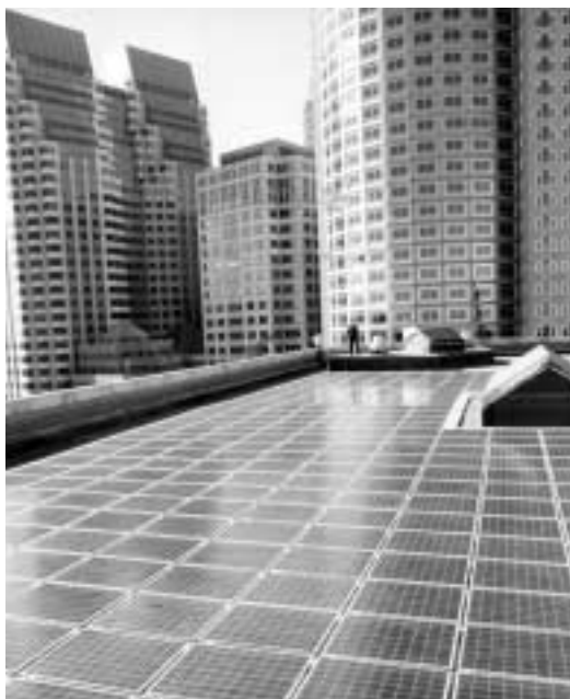
A 28-kW AC photovoltaic system consisting of 372 PV panels at the GSA Williams Building in Boston, Massachusetts
