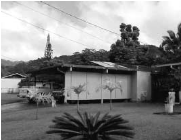
Large solar water heating project at the Kia'i Kai Hale housing area in Honolulu, Hawaii
