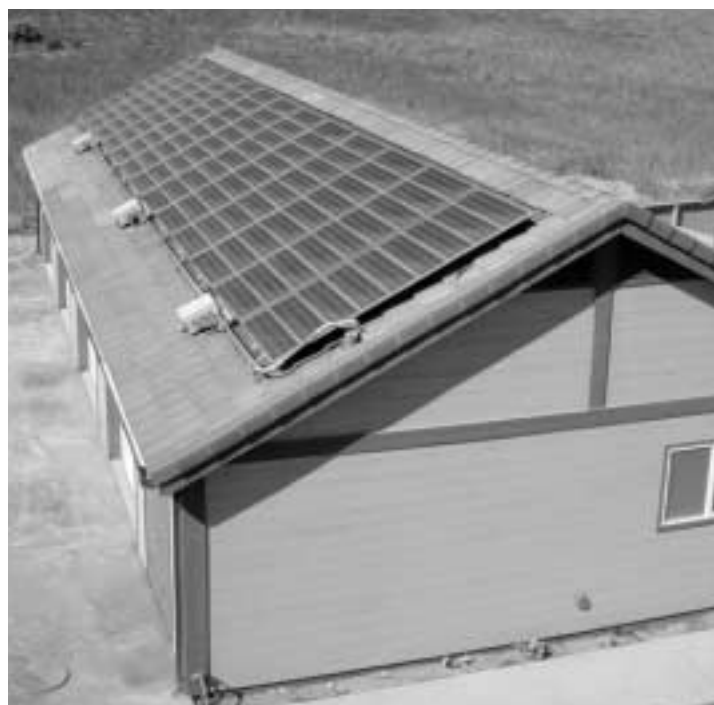
A 6.4-kW photovoltaic array on Santa Rosa Island, Channel Islands National Park, California
