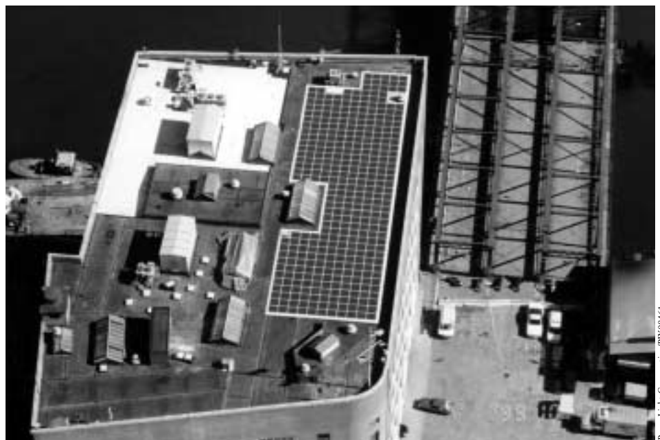
A 28-kW AC photovoltaic system consisting of 372 PV panels at the GSA Williams Building in Boston, Massachusetts
