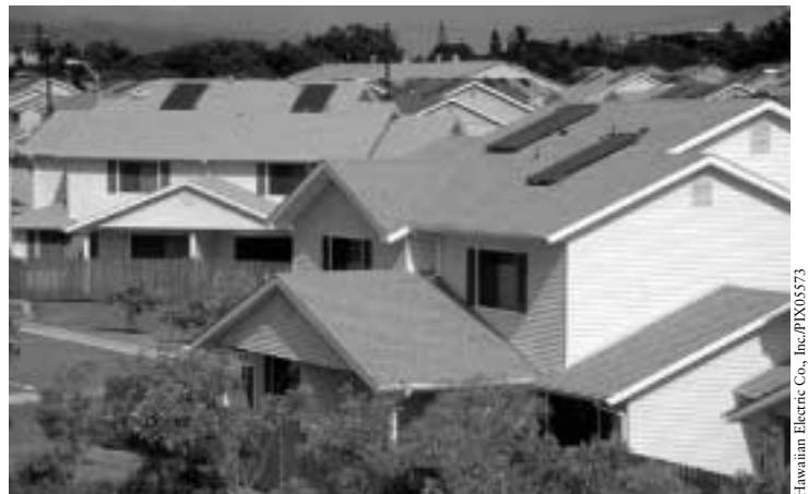
Solar water heating units at Moanalua Terrace in Oahu, Hawaii
