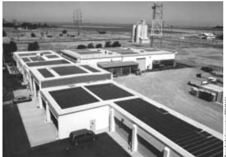
2-kW prototype photovoltaic (PV) unit at Western Area Power Administration facility in California
