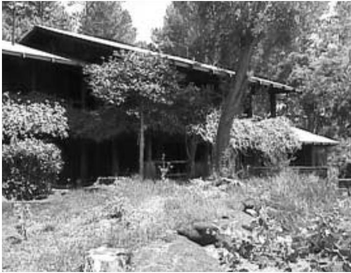
Photovoltaic system at Ainahou Ranch, a historic building located in Volcanoes National Park in Hawaii
