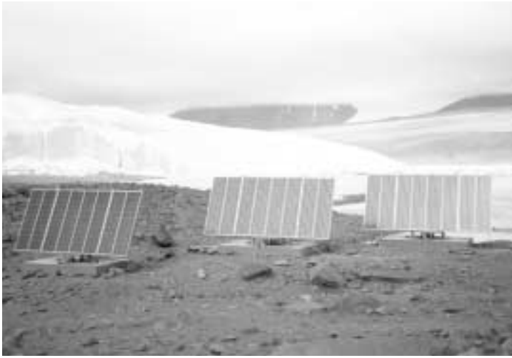
A 1.2-kW photovoltaic system at Lake Hoare, Antarctica
