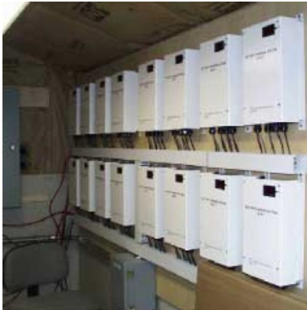
**Figure 1. Battery-Charging System**
