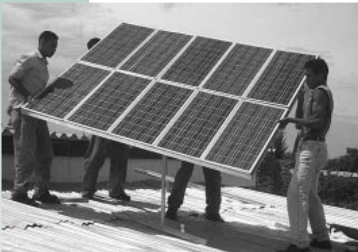
Figure 3.1. Multiple modules can be connected for larger energy needs.
