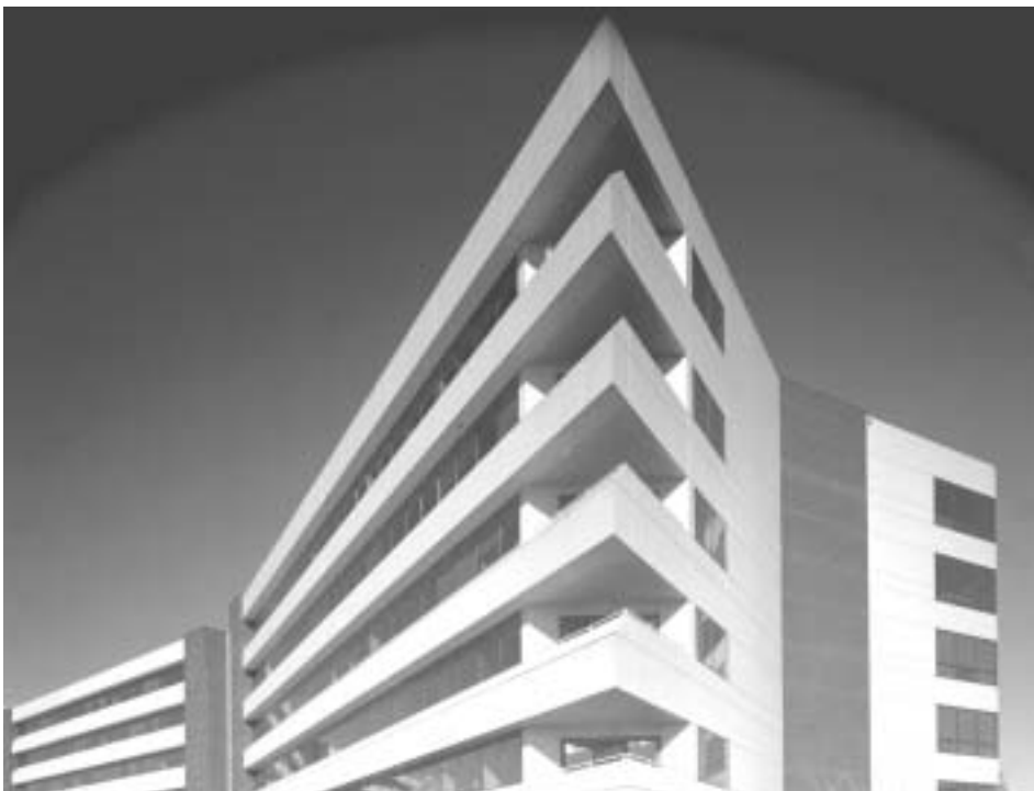
This building has differentiated façades—broad overhangs for shading on the south side and no overhangs on the north side.
