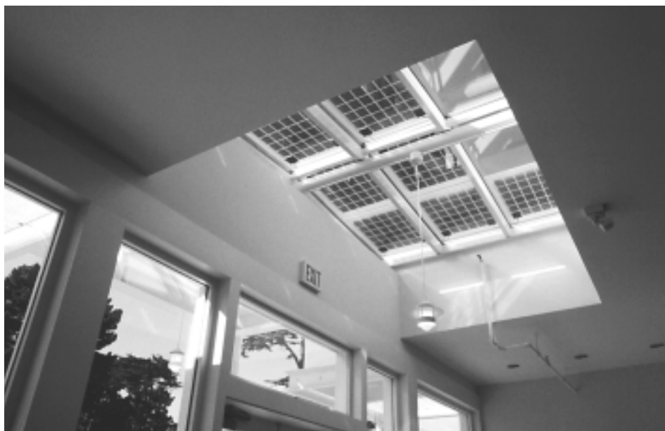
A skylighted entryway that also demonstrates the integration of photovoltaics at the Thoreau Center for Sustainability at Presidio National Park, California.
