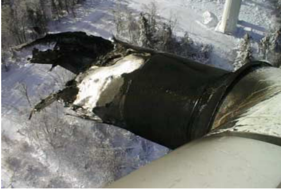
Figure 5. Blade damage at Searsburg, VT
