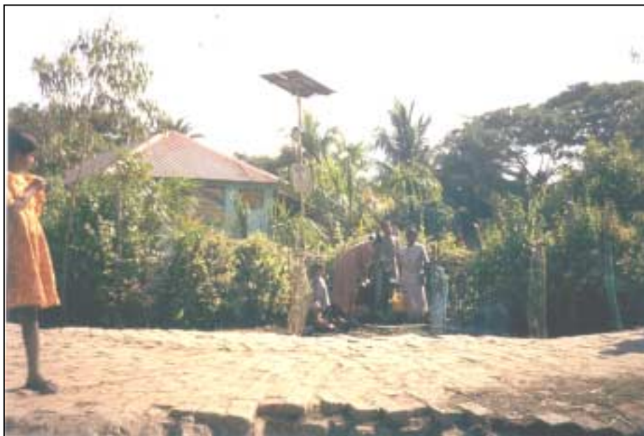
Figure 8 Streetlight and lighting systems in youth club Satjelia
