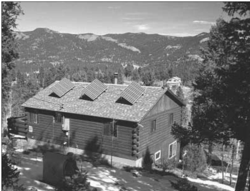
Terry Schuyler, NREL/PIX07679
