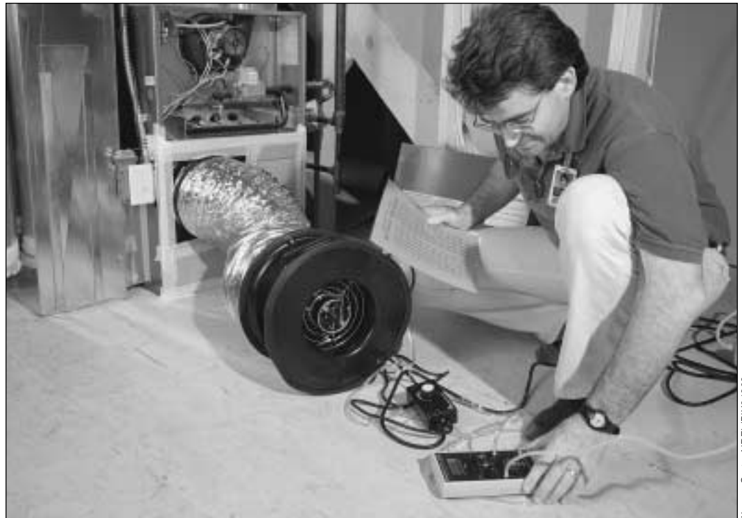
A home energy rating inspection sometimes involves a duct blaster test, which measures air leakage in the ductwork.
