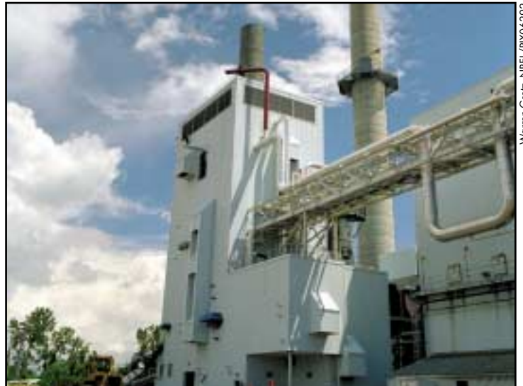
A high-throughput biomass gasifier converts biomass into gas for electric power generation.
