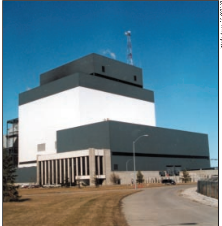
Alliant Energy's Ottumwa, Iowa, Generating Station
