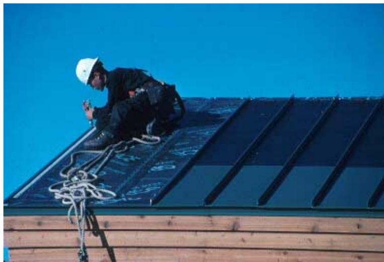
**Figure 5. Installation of the Photovoltaic Roof**
