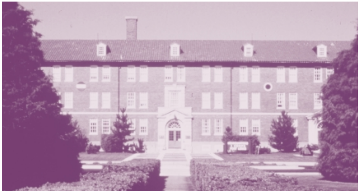
HEADQUARTER I CORPS IS ONLY ONE OF THE MANY BUILDINGS AT FORT LEWIS IN TACOMA, WASHINGTON, THAT WAS MADE MORE ENERGY-EFFICIENT THROUGH FEMP AND SEP SPECIAL PROJECTS.
