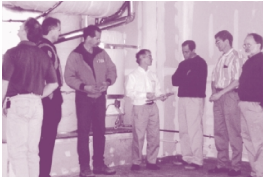
THE THOROUGH INSPECTION OF WATER HEATERS AND OTHER MAJOR APPLIANCES IS CRUCIAL IN DETERMINING WHICH ENERGY-EFFICIENT ADJUSTMENTS ARE REQUIRED IN NEW AND EXISTING BUILDINGS.
