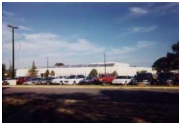
Fig. 3: A large, solar water-heating system is being refurbished in this two-phase project in New Mexico.
