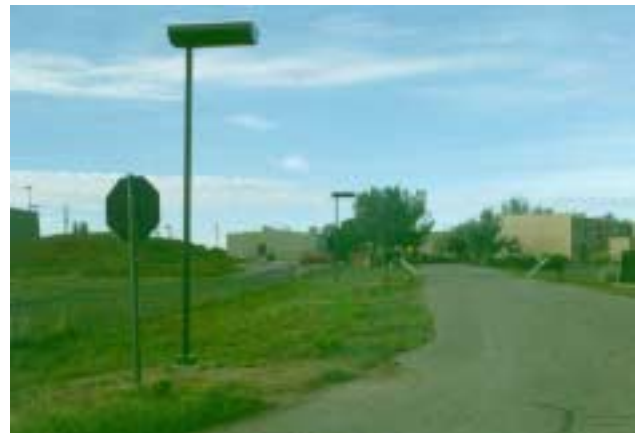
Fig. 1: Photovoltaic-powered lights, like the ones installed at an Indian Health Service facility in New Mexico, are listed on the GSA Solar Supply Schedule.
