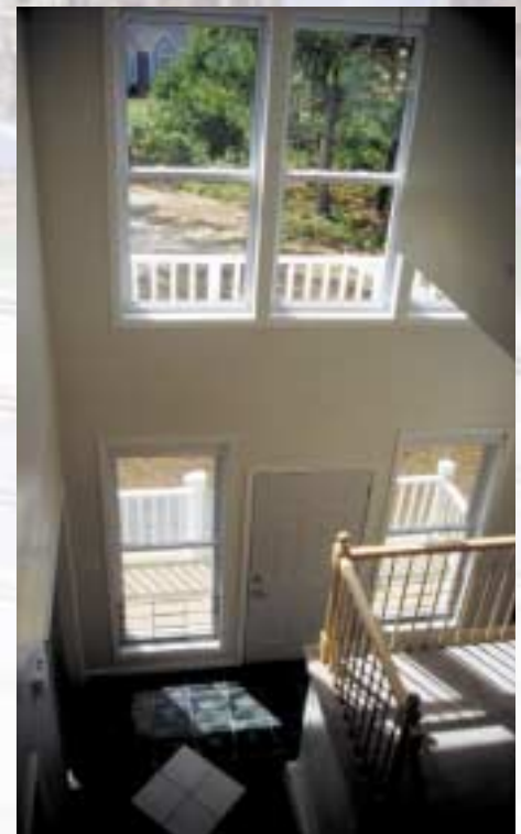
Large south-facing windows provide direct solar gain to the interior of the home, while dark-colored tile absorbs and holds heat from the sun.
