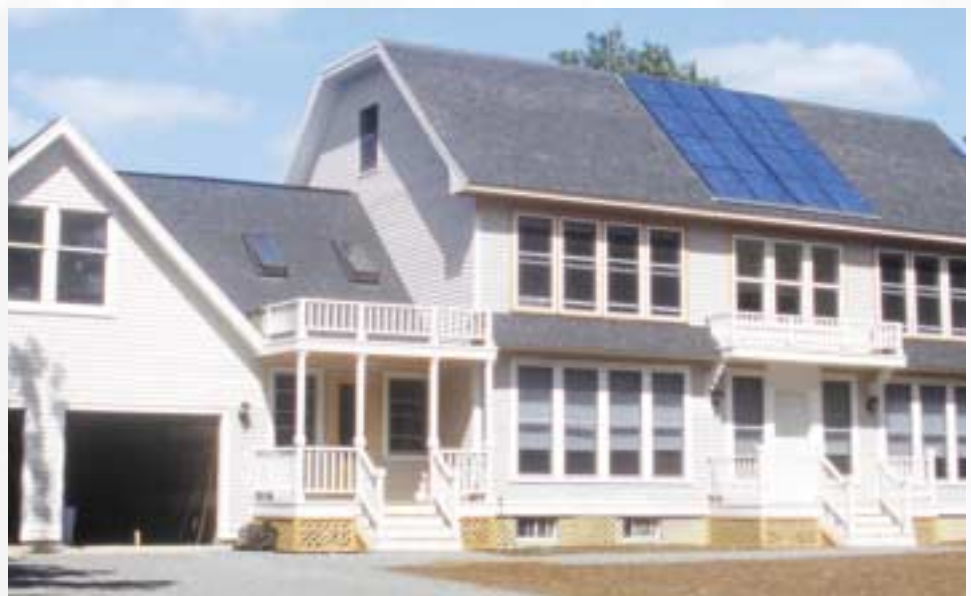
Solar energy meets 78% of this home's heating needs. The 16 PV modules, which can be factory-installed or site-mounted on the roof, provide virtually all of the home's electricity. (Manufacturer: AvisAmerica homes.)
