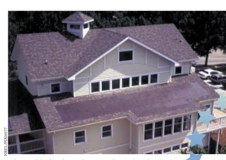
The PV shingles shown here on a house in Atlanta, Georgia, won Popular Science magazine's grand award for "What's New in Environmental Technology." The PV shingles cover the inner portion of the lower roof section.
