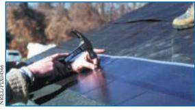
Thin-film PV shingles installed on building rooftops can take the place of conventional asphalt shingles and generate electricity.
