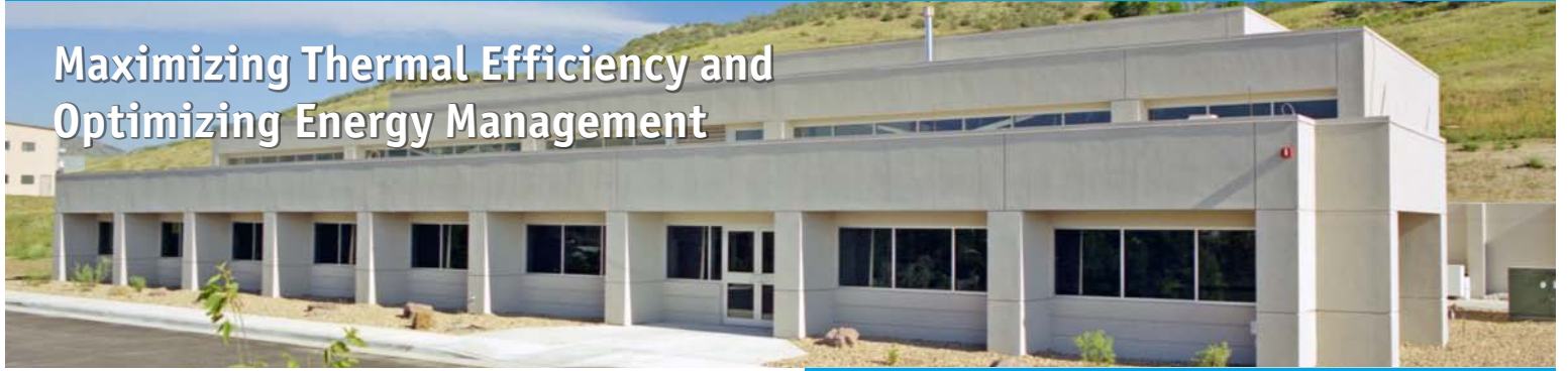
Photo by Warren Gretz, NREL/PIX 01014
