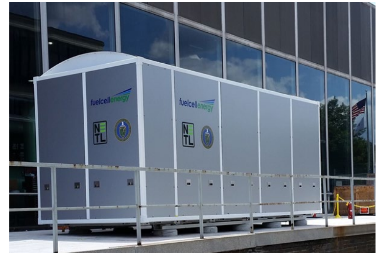
200 kWe integrated SOFC Power System: ~2,000 full-scale cells (Photo courtesy FuelCell Energy)
