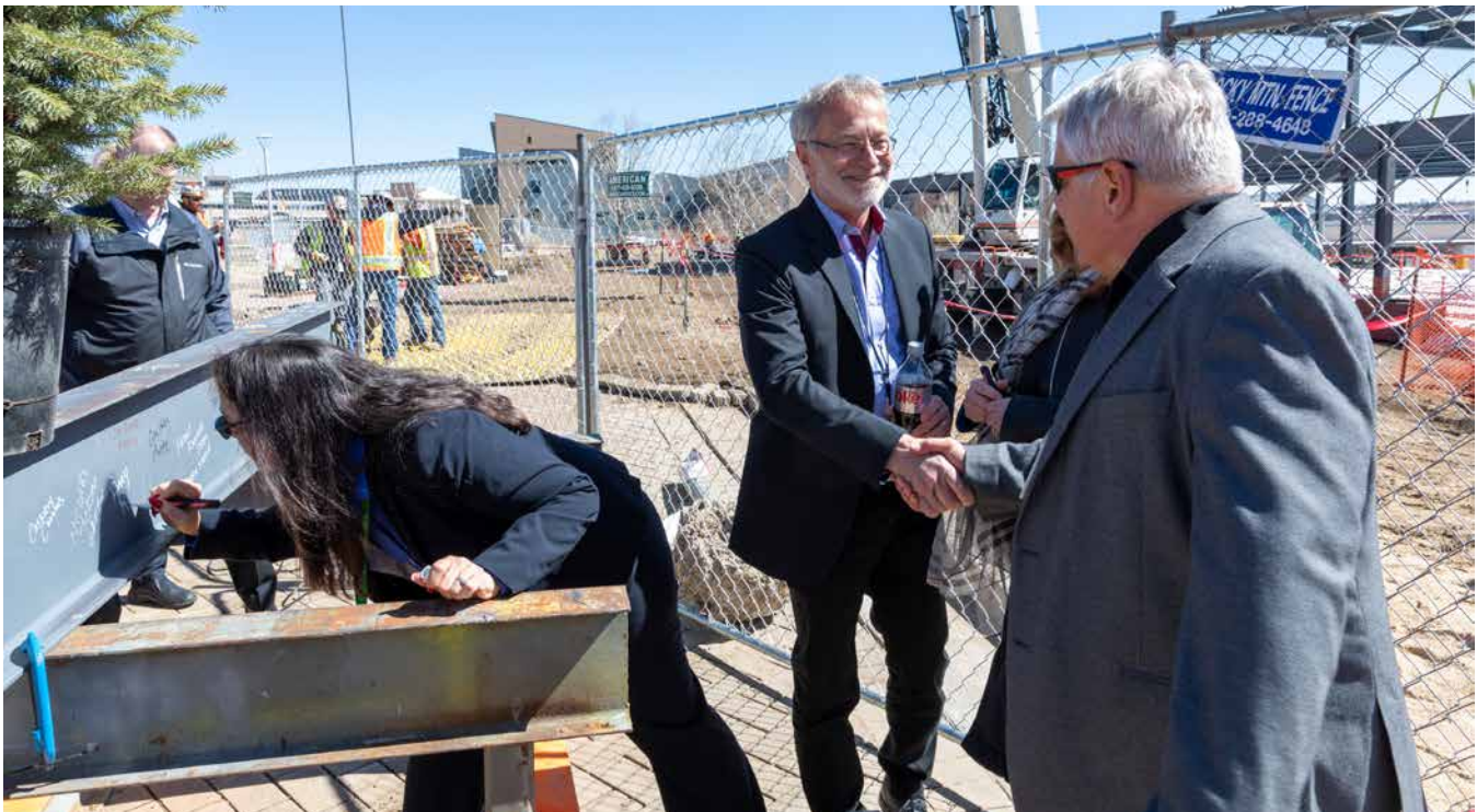
Martin Keller (center) greets Associate Lab Director for Materials, Chemical, and Computational Sciences Bill Tumas, in March 2022, while Amy Read (left) of the U.S. Department of Energy's Golden Field Office signs the final beam during the topping-out celebration for the Research And Innovation Laboratory (RAIL) on NREL's South Table Mountain campus. Photo by Werner Slocum, NREL 66777
