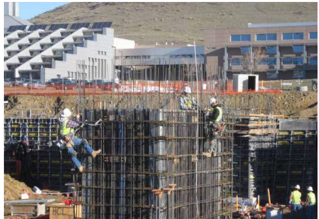
NREL’s Research Support Facilities (RSF) under construction. Photo by Carl Cox, NREL 16282
