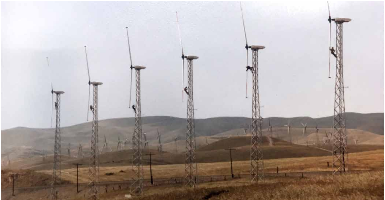
Blade washing crews working on ESI-54 wind turbines on Jess Ranch in Altamont Pass, California in 1985. Photo by Walt Musial, NREL
