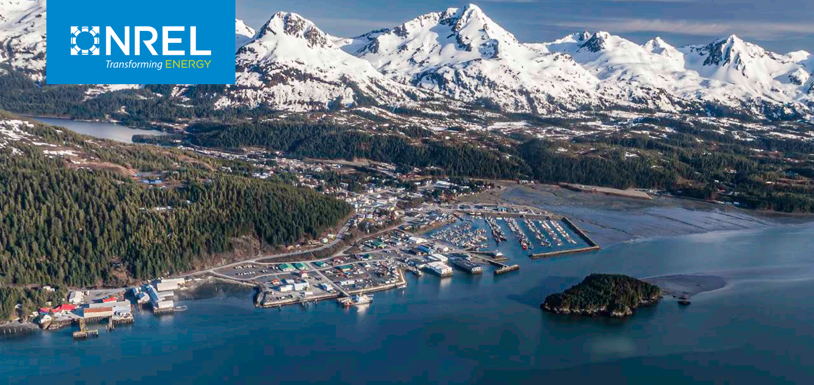
Cordova, AK, a coastal city and microgrid that delivers power to 2,700 residents. Photo from iStock, 1282751408
