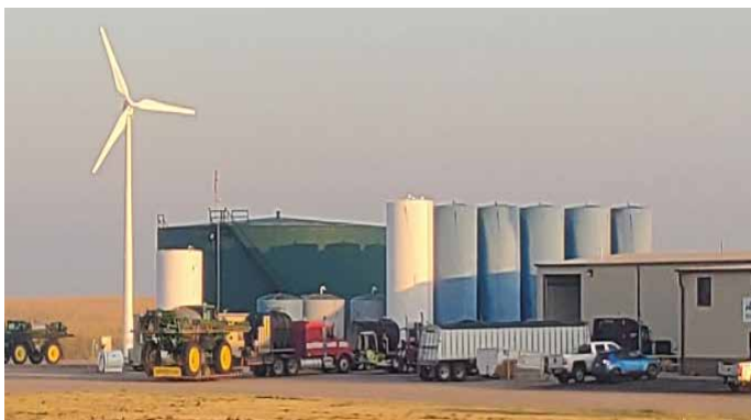
An Eocycle EOX S-16 Model 25-kilowatt turbine installed at Nutrien Ag Solutions, a company dedicated to helping growers achieve high crop yields sustainably. Photo from Eocycle
