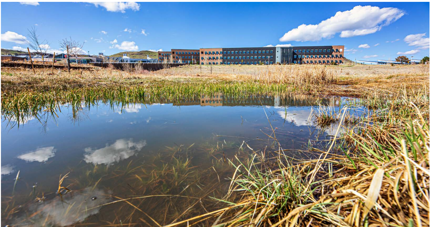
The Central Arroyo Detention Basin near the parking garage on the STM Campus was created to direct stormwater away from campus. The detention basin also provides habitat for various species. Photo by Werner Slocum, NREL 64473
