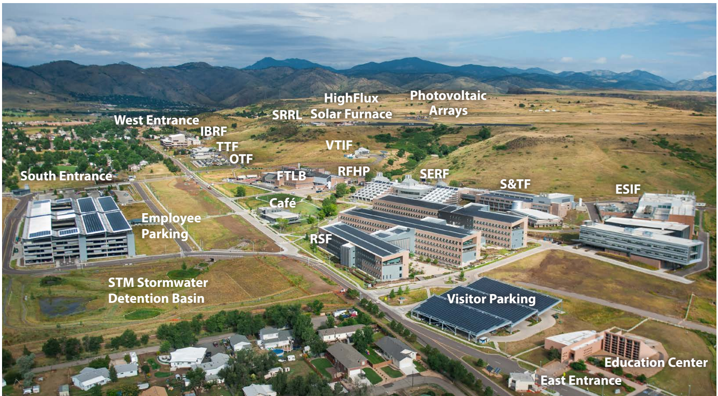
An aerial view of NREL's STM Campus. Photo by Dennis Schroeder, NREL 30709
