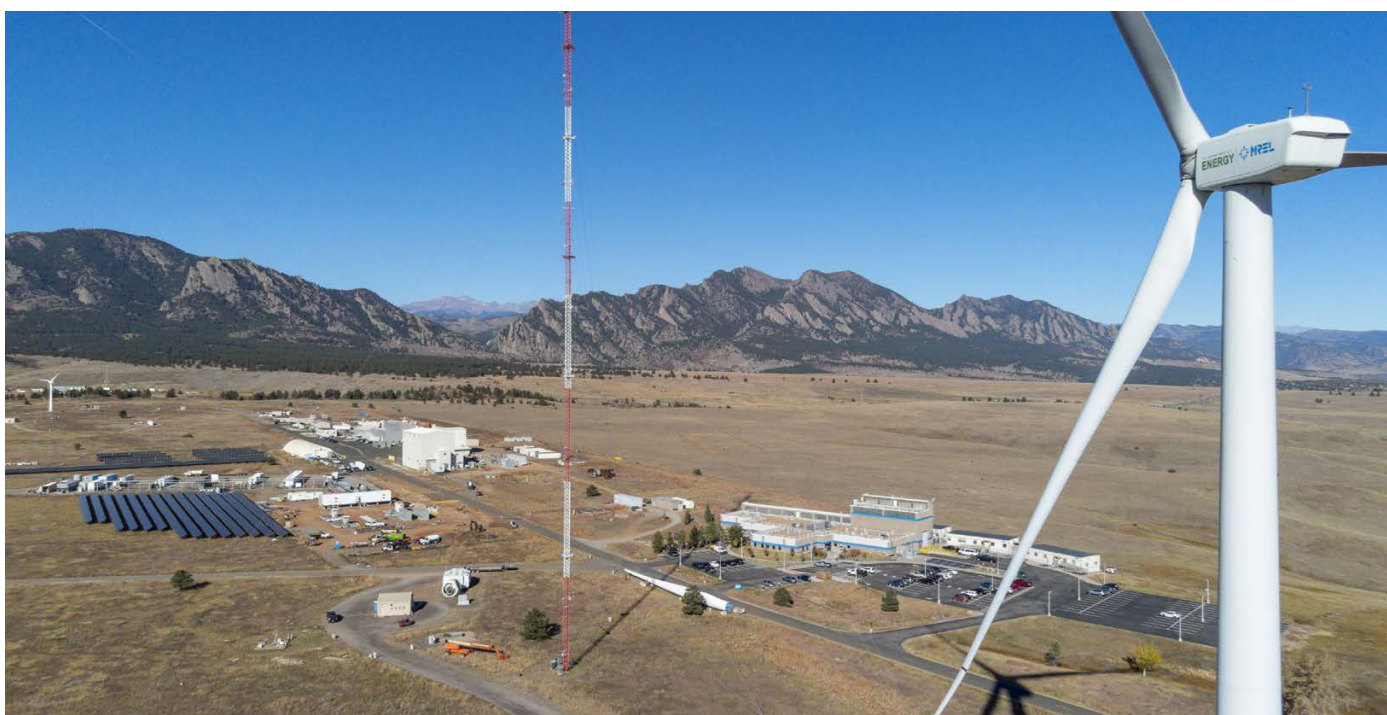
Overall aerial view of the Flatirons Campus looking west. To the right is a 1.5-megawatt turbine. Photo by Josh Bauer and Bryan Bechtold, NREL 73093
