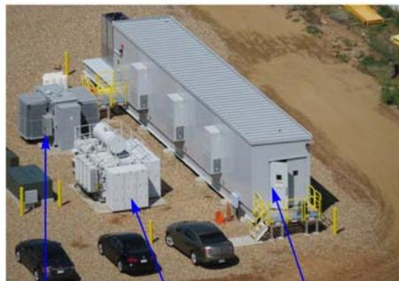
Grid-side transformer    Output transformer    ARU + 4 NP-VSC in parallel
