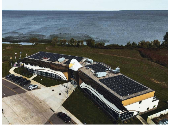
A 70-kW solar array at the Red Lake Band of Chippewa Indian Tribal government center. Photo by Robert Blake, Native Sun
