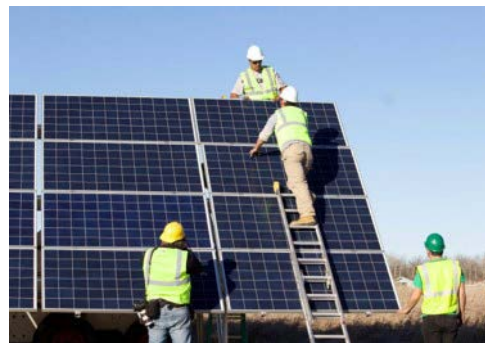
Leech Lake Tribal College students gain hands-on workforce experience installing a solar PV array. Photo by Eugene Strowbridge, Leech Lake Band of Ojibwe
