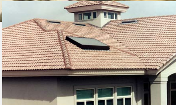
Photo by Warren Gretz, NREL 25967
