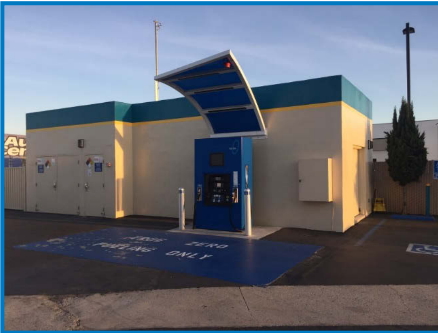
FirstElement Fuel, Costa Mesa, CA. Photo: NREL
