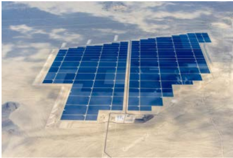
Figure 6. Aerial photo of First Solar’s 300-MW PV power plant. Photo from First Solar
