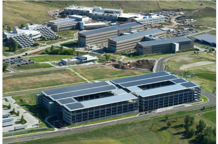
Renewable energy power is produced from photovoltaic panels on the garage rooftop and on the south façade.
