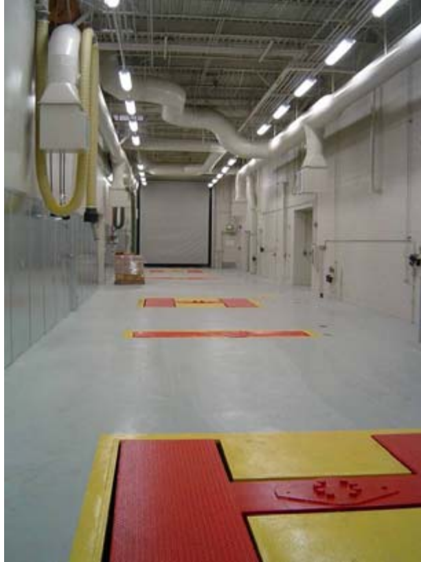
Figure 10. Modified maintenance bay at AC Transit
