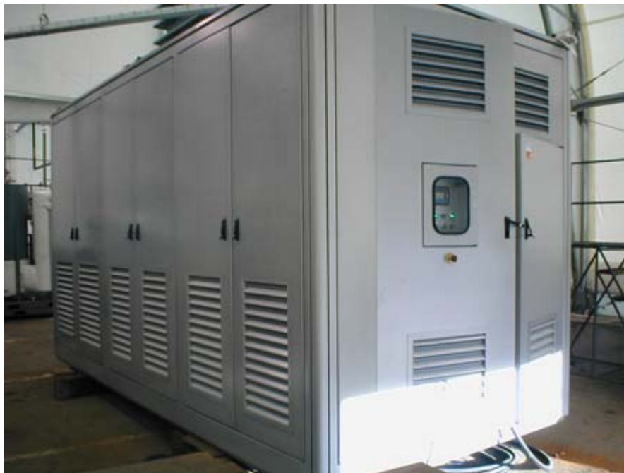
Figure 6. Reformer train #1 at Chevron – AC Transit Hydrogen Energy Station (75 kg/day)
