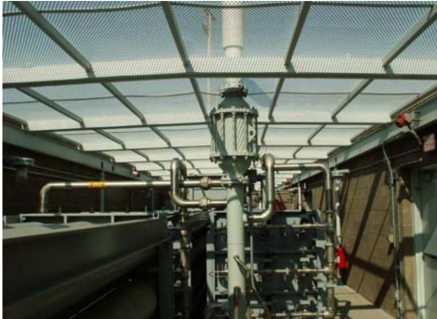
Figure 7. Cascade hydrogen storage vessels at AC Transit station
