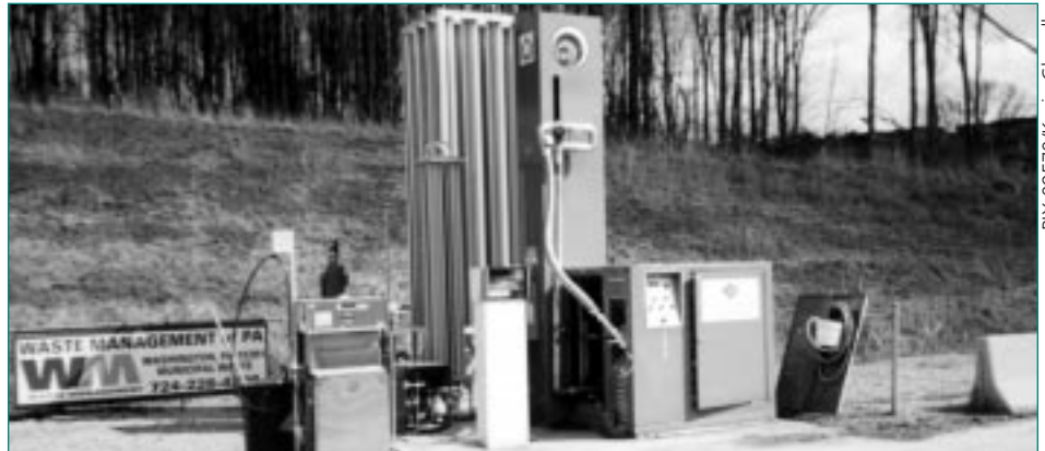
Figure 2. LNG fueling station with added LCNG components
