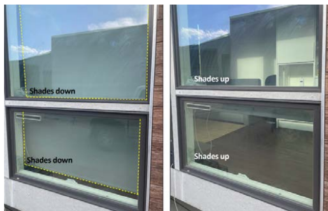
Figure 4. Dynamically controlled shading, triggered by demand response events at the NREL campus in Golden, CO. Source: NREL.
